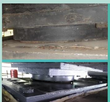
Clockwise from top left; Rust jacking of sliding plates; Typical guide damage; Reinstating guides; Cleaned and polished bearing.
