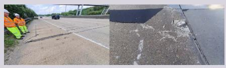
Exposed concrete sections which buckled due to temperature. Left photo – 21/07/2021 M25 B Carriageway MP 56/4+70. Right photo – 23/07/2021 M25 A Carriageway MP 145/4
